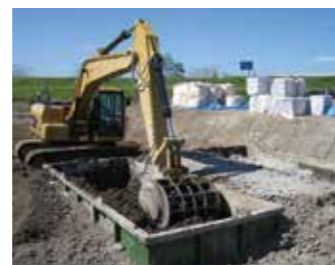
Reutilization of tsunami debris via fiber-cement-stabilized soil method.
