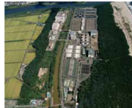
Minami Gamou Water Purification Center, Sendai.
