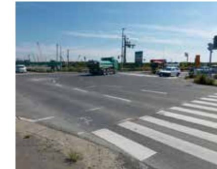
Before the installation.
