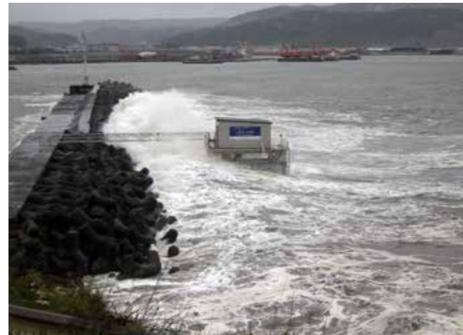
Power generation during a typhoon
