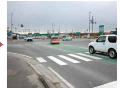
After the installation
