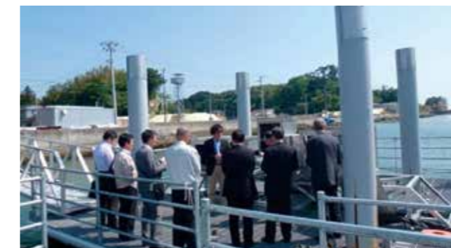
Oceanic tidal power generation facility
