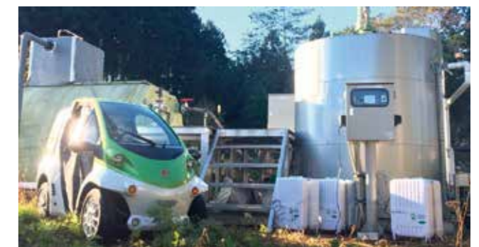
Charging a small electric car with produced biogas fuel.
