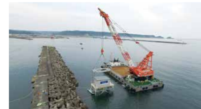
Installing wave power generators
