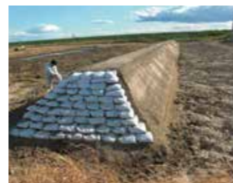
Dike constructed with fiber-cement-stabilized soil.
